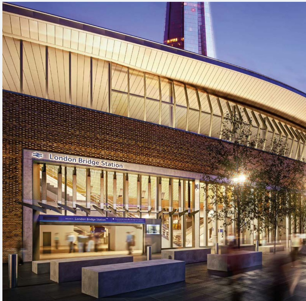
Contract value: £1b Type of work: Redevelopment of Victorian railway station
